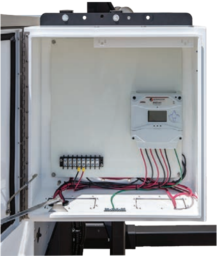
Control box wired and ready for installing electronics
